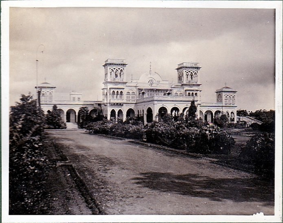
A Parsee mansion on the Bund Garden Road.
